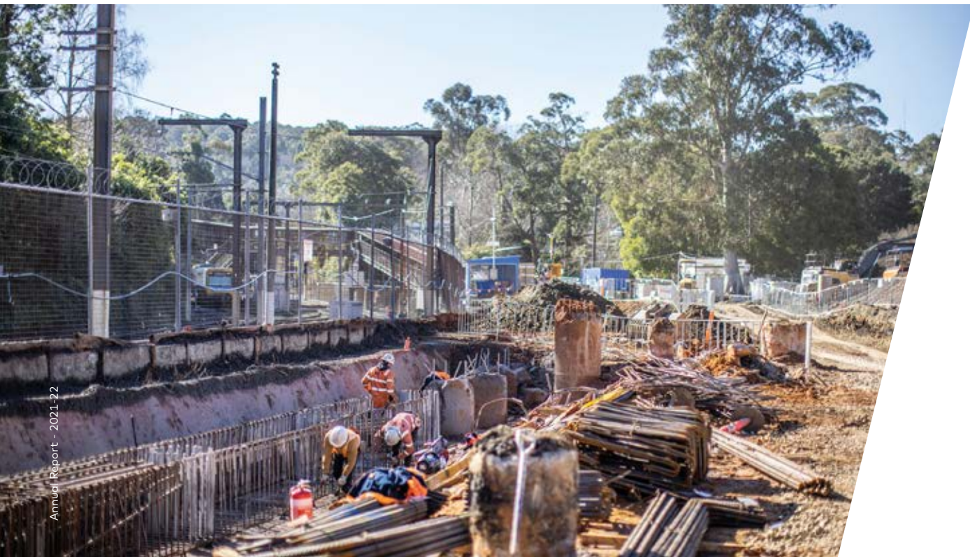
Piling works at Belgrave Station
