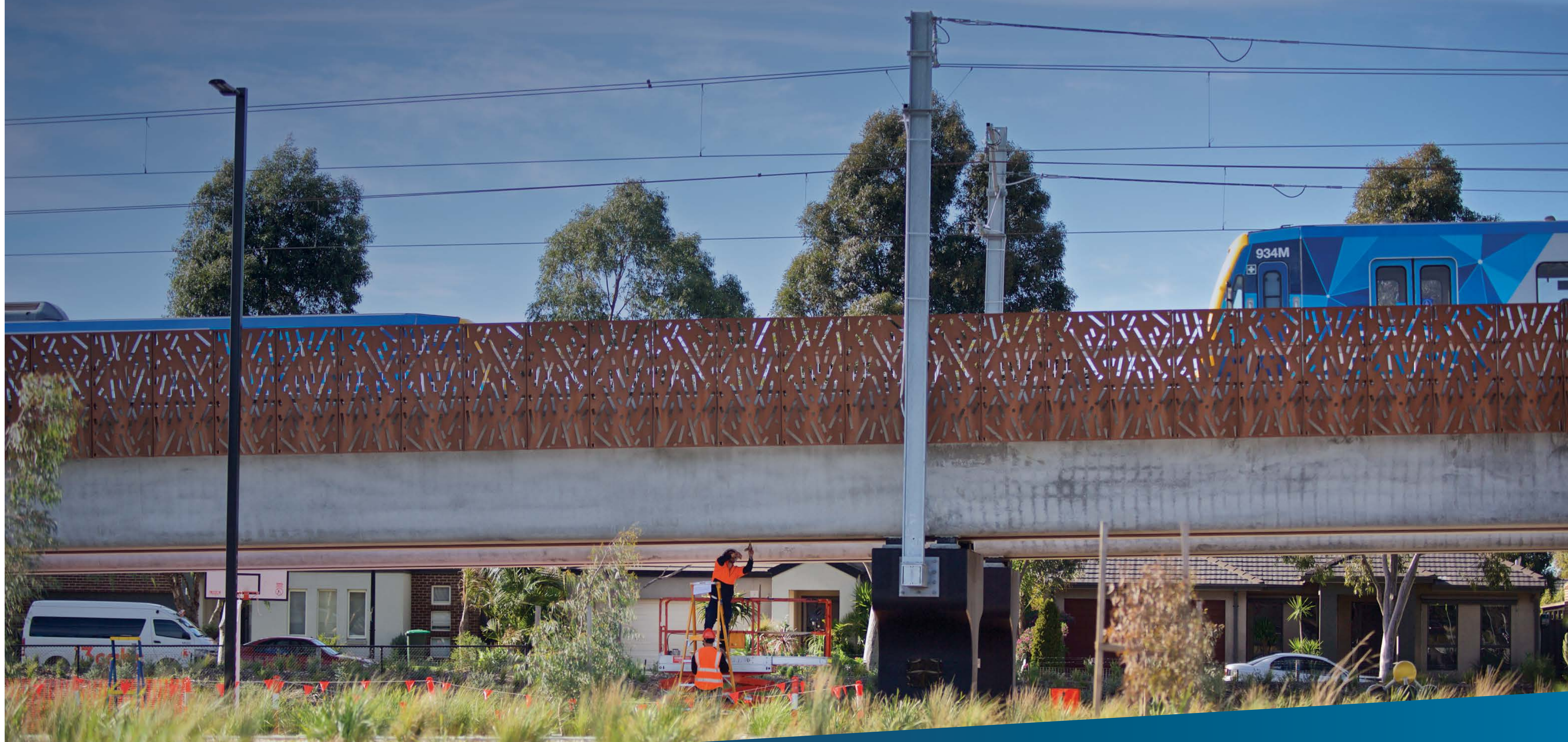
Installation at Hawkstowe Station
