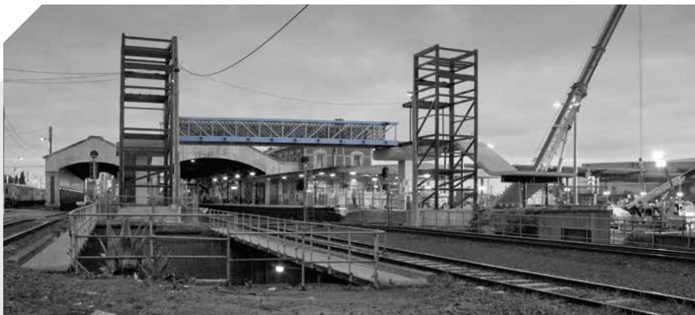
Geelong Station night works.
