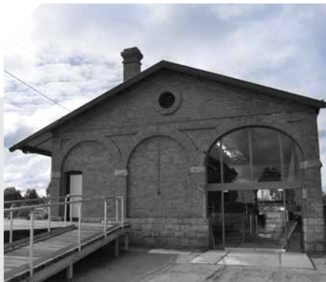
The refurbished Chiltern Station goods shed.
