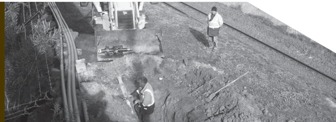
Above: VicTrack has installed 1220 km of fibre optic cable along Victoria's rail corridors.
