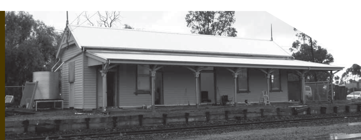
Above: Restoration works nearing completion at Wycheproof Station, built in 1887.
