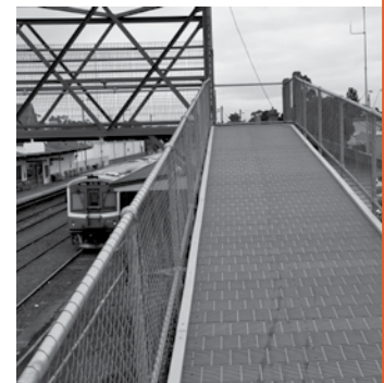
Traralgon station footbridge was resurfaced during the year
