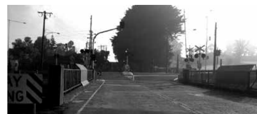
Lardner’s Track level crossing upgrade
