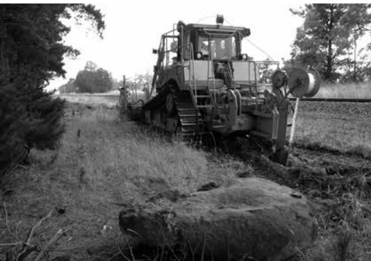
Installing fibre for the Victorian Fibre Strategy near Boorcan.
